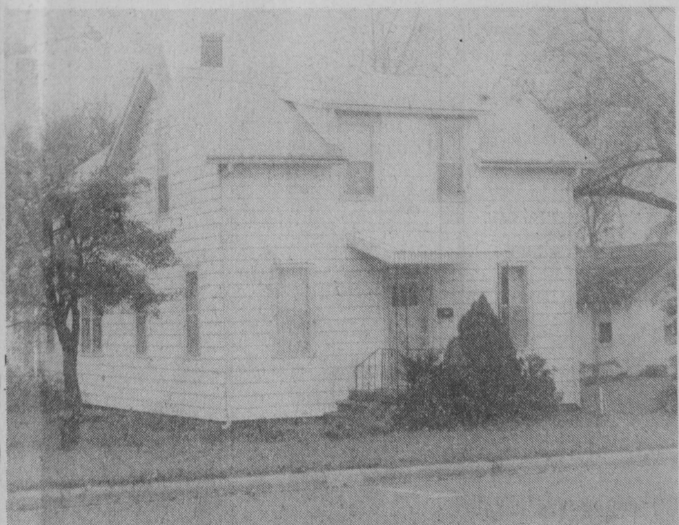
THIS RESIDENCE overlooking Tawas Bay was owned by John Mark. When he and his family moved there in 1899, the bridge near the mouth of the Tawas River had been
