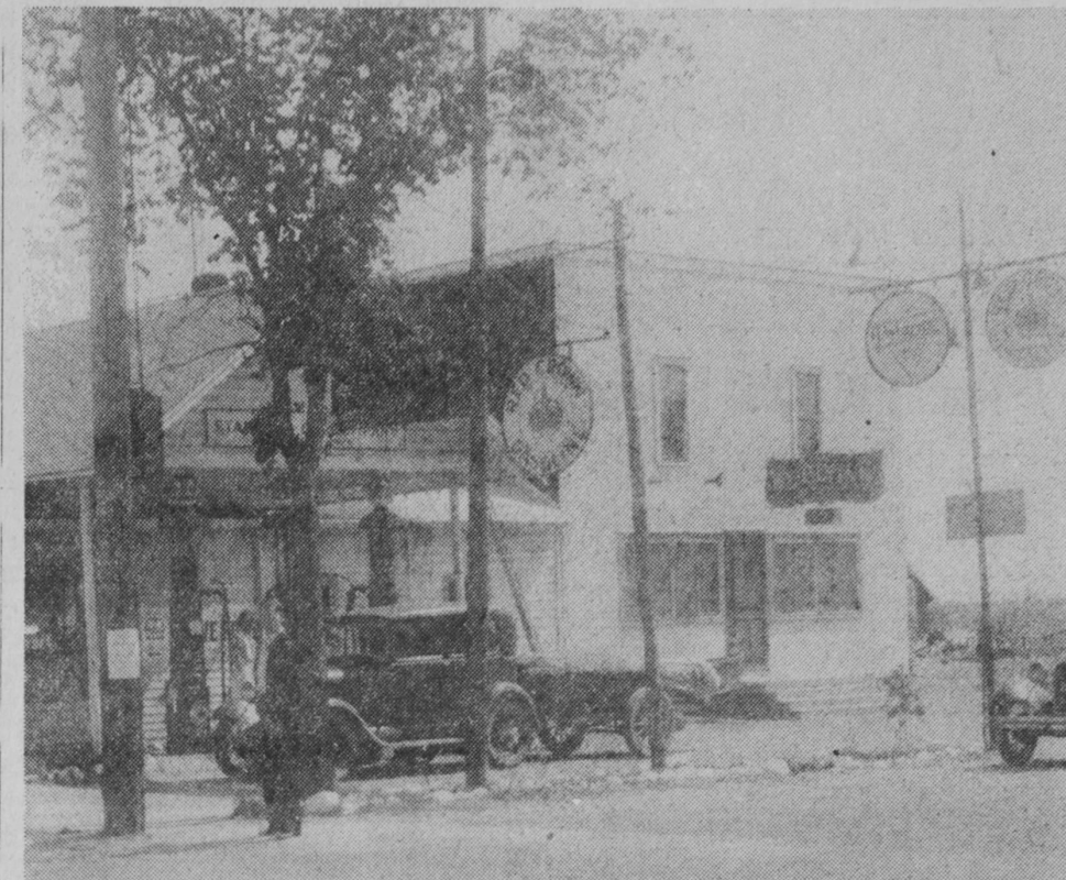
GASOLINE SERVICE STATIONS were established soon after state trunklines were designated in this region. This station was located at Hale when M-65 was established in the early 1930s. This route followed an older road through Twining and Whittemore and proceeded in a northerly direction through Hale after establishment of the Huron Shore Road.
