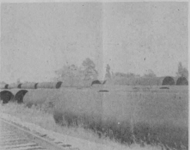
AN EXTENSIVE operation for preparing the pipes was located at the West Tawas yard of the Detroit and Mackinac Railway in Tawas City. After processing, a water-tight bulkhead was affixed to each end of the pipe. Launched and floated under the US-23 bridge into Tawas Bay, a tugboat towed the long sections to Whitestone Point.—Tawas Herald Photos.
