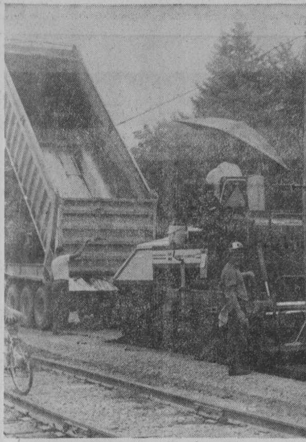
WORK was completed as scheduled last week on a street blacktopping program in Tawas City. Central Paving Company, contractor, was at work on Court Street in the above photo.—Tawas Herald Photo.
