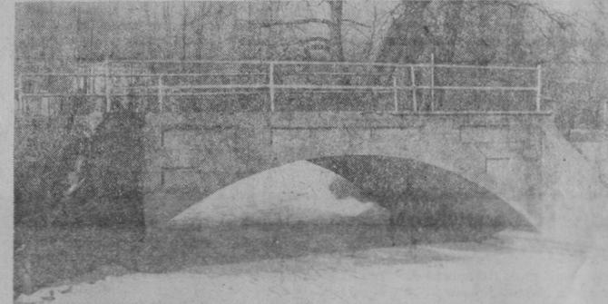
THIS CONCRETE ARCH BRIDGE spanning Dead Creek was constructed in 1912 and its abutments have deteriorated. Emergency repairs were made to the structure last year,
