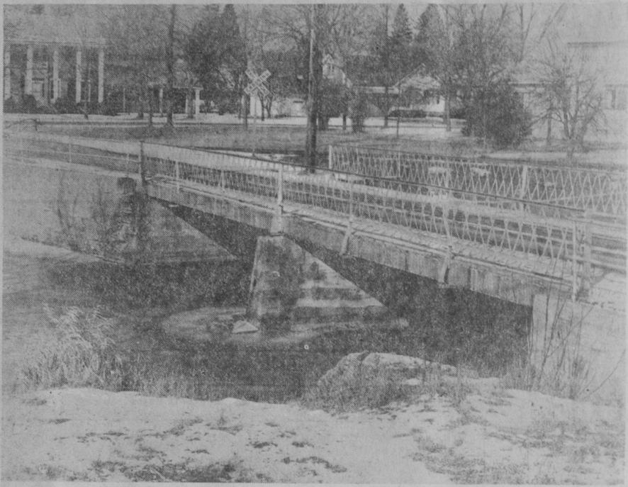
THE WHITTEMORE STREET BRIDGE has deteriorated rapidly in recent years, as evidenced by crumbling concrete on the southwest abutment shown in this picture. The
