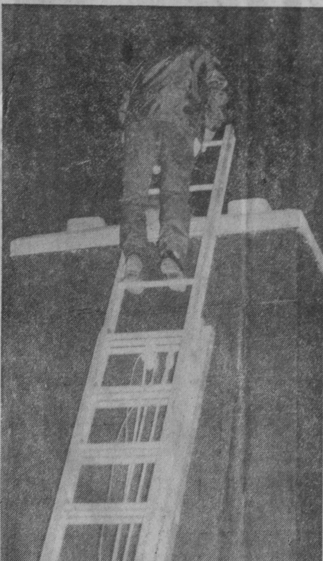
SANTA CLAUS was not the only one to climb chimneys over Christmas. This Tawas City volunteer fireman used a ladder to check this chimney for a burnout when firemen were called to the scene at a Tawas City dwelling. The department suggests that home owners check chimneys and remove any accumulation of creosote left from burning wood.—Tawas Herald Photo.
