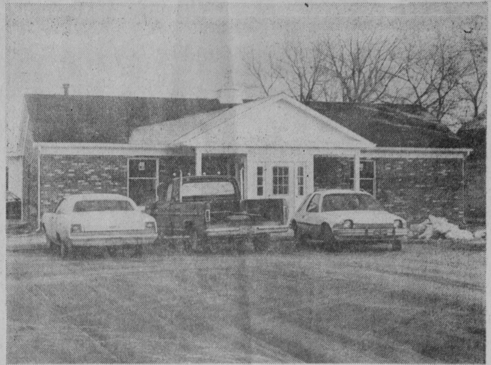
A RIBBON-CUTTING ceremony is to be held Wednesday morning, 8:45 o'clock, at the new Hale branch office of Peoples State Bank of East Tawas. Ground was broken for the structure in the fall and contractor for
