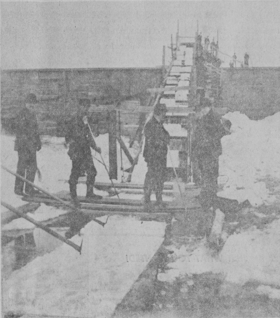
A MECHANIZED CONVEYER is being used here to move ice directly from the bay to a large shed on Tawas Point. Tawas Bay ice was noted for its purity and found a ready
