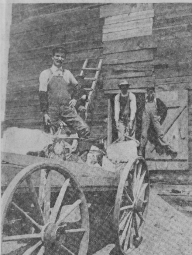
BUILDINGS insulated with sawdust were used to store ice. The wooden frame structures had double walls and the space between the walls was filled with sawdust. In packing the ice, each layer was protected by a covering of sawdust, which had to be washed off before delivery.
