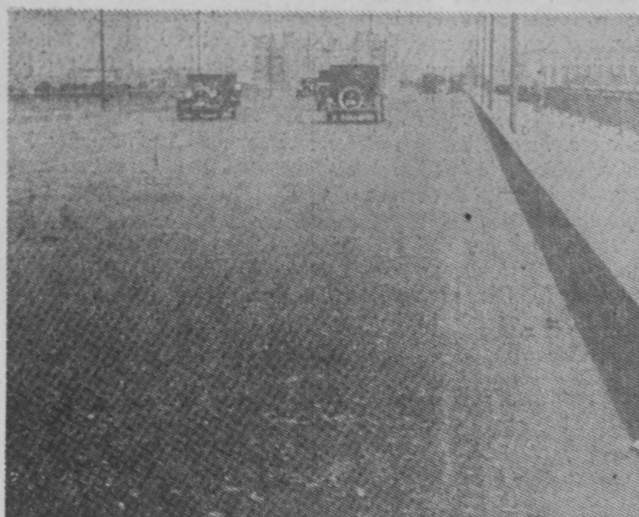
ONE OF THE achievements of Michigan during the 1920's was construction of Wider Woodward Avenue from Eight Mile Road to Pontiac, the first modern divided highway in the country. Its designer was Leon Belknap, who was born at Whittemore and became chief engineer of the Oakland County Road Commission at Pontiac.
