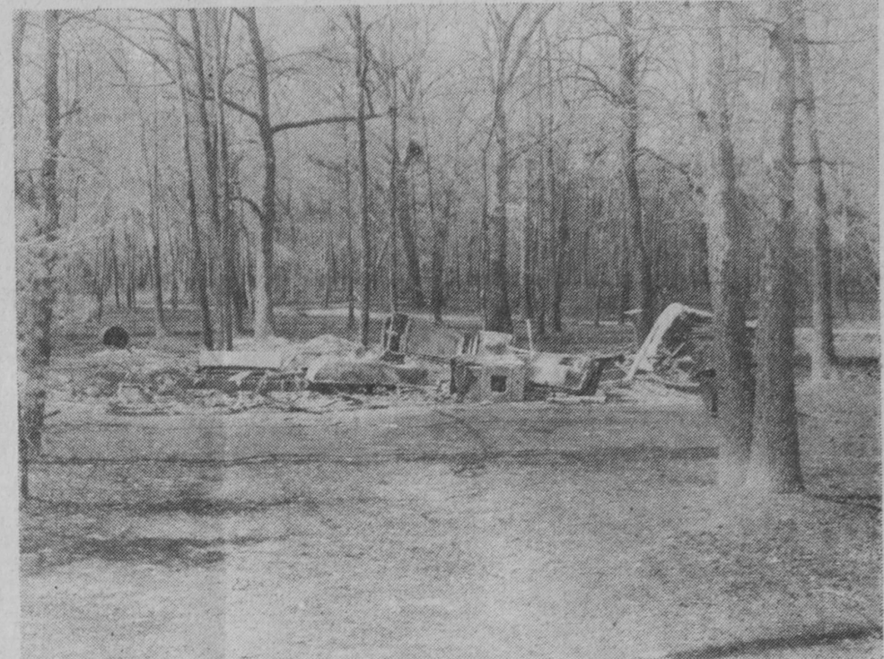
DAMAGE to private property in a 300-acre fire which struck near Little Island Lake was amazingly light. This mobile home in cabin and a garage were damaged, but cabins tied around the lake escaped damage.—Tawas Herald Photo.
