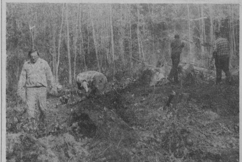
THE TAWAS CITY Department of Public Works crew was busy Monday felling trees which were in the path of a road to the new industrial park west of Ninth Avenue. Sixth Street is being extended into the 40-acre
