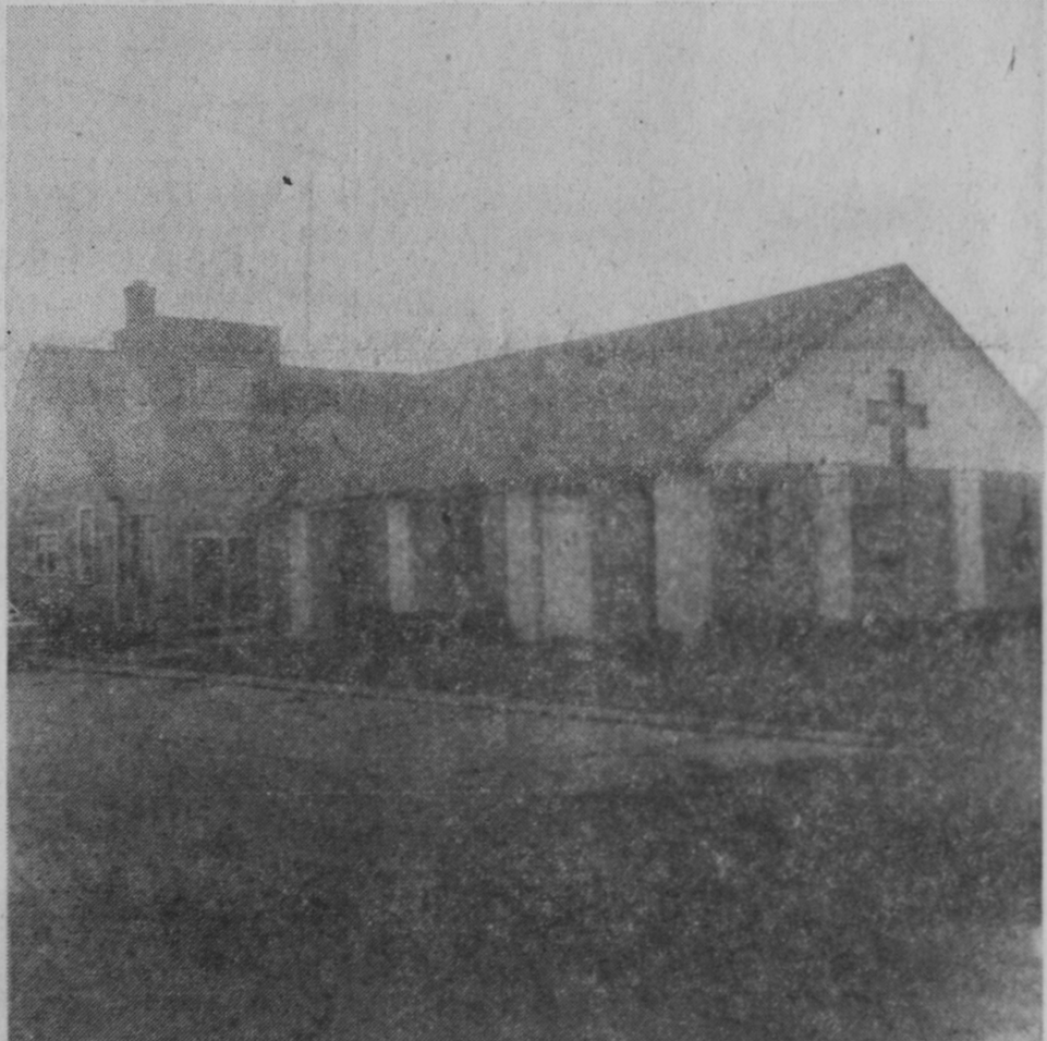
A NEW ADDITION is being constructed at the rear of St. Paul's Lutheran Church, Hale, above. Work on the project is expected to be
