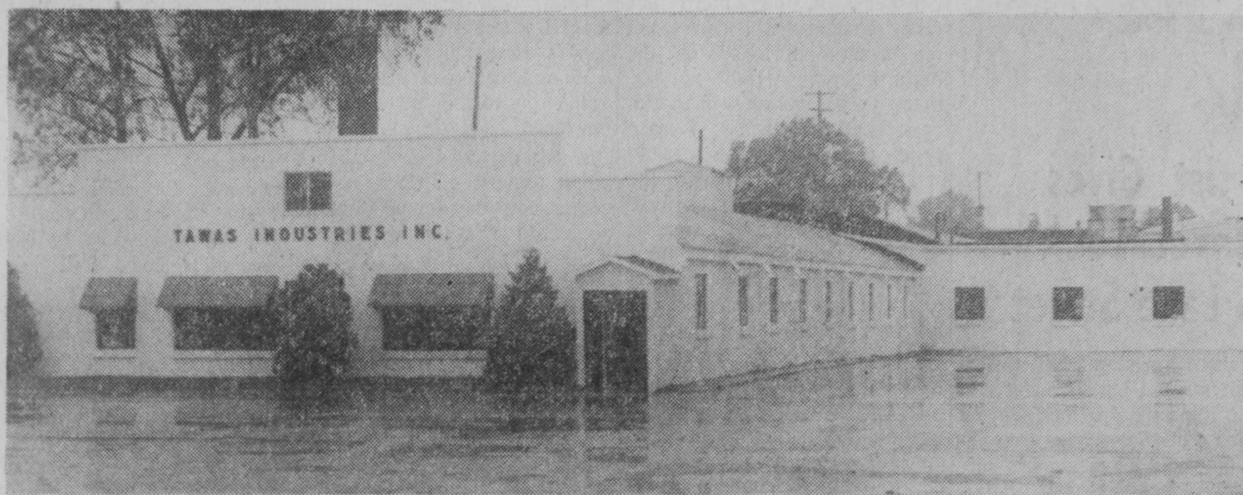
A TRANSACTION is to be completed later this week whereby this industrial building presently occupied by Tawas Industries, Incorporated, will become the new location of Brugger's Foodland, along with possibly two mercantile stores.
