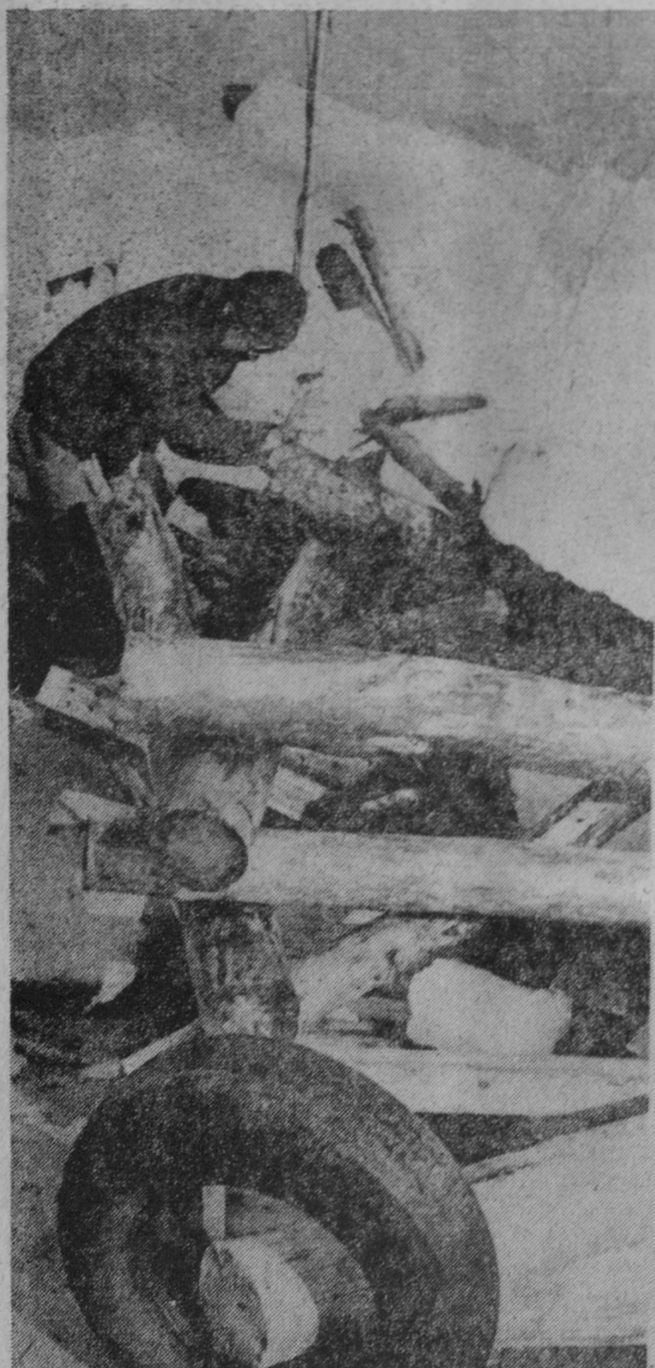
A SPECTATOR views the remains of a wooden dock which was in the path of the ice floe. It was broken apart and tossed on the shore.—Tawas Herald Photo.
