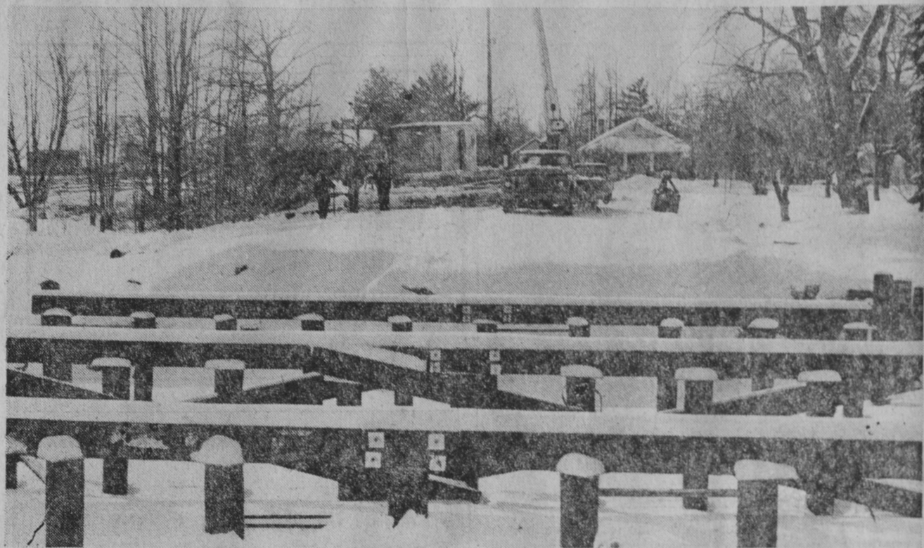
THIS WINTER is going down as one of the coldest in recent years, the first 24 days of January registering temperatures well below normal for that month. Following last week's storm which dumped about nine inches of snow on the area, the temperature dropped to 20 degrees below zero Thursday morning. One of the coldest jobs in the area is being performed by workmen of Great Lakes Contractors of Warren, who are replacing two bridges in Tawas City. The
