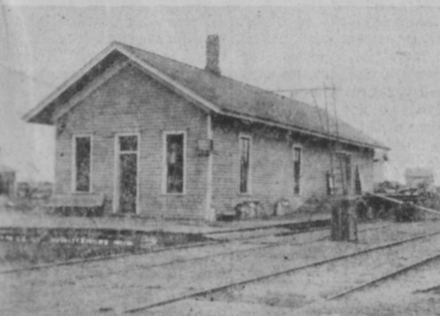
THE DETROIT AND MACKINAC Railway Depot at Whittemore is pictured here in the early 1900s. The building was later moved, after abandonment of the Prescott Division, and converted into a dwelling.
