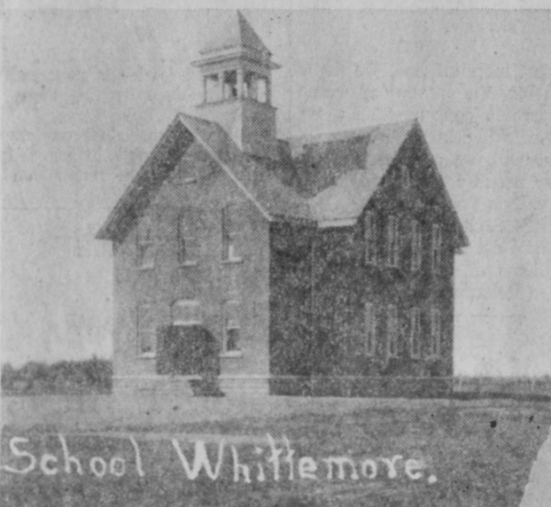
THIS SCHOOL BUILDING was constructed in 1907 and the first year of school was held beginning in September of that year "with Mr. Lisle and Florence Schroyer (Curtis) as teachers." An addition was later made to the building and it was used as an elementary school after consolidation of the Whittemore-Prescott Area School District. It was razed about 10 years ago.
