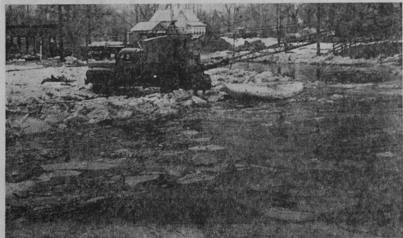
ANNUAL SPRING BREAKUP of ice in Dead Creek came last Thursday and this dragline of the Tawas City Department of Public Works was at work in the fog clearing an ice jam near the railroad bridge. This scene usually is a signal that spring is not far behind, but several weeks more of winter weather can be expected.—Tawas Herald Photo.
