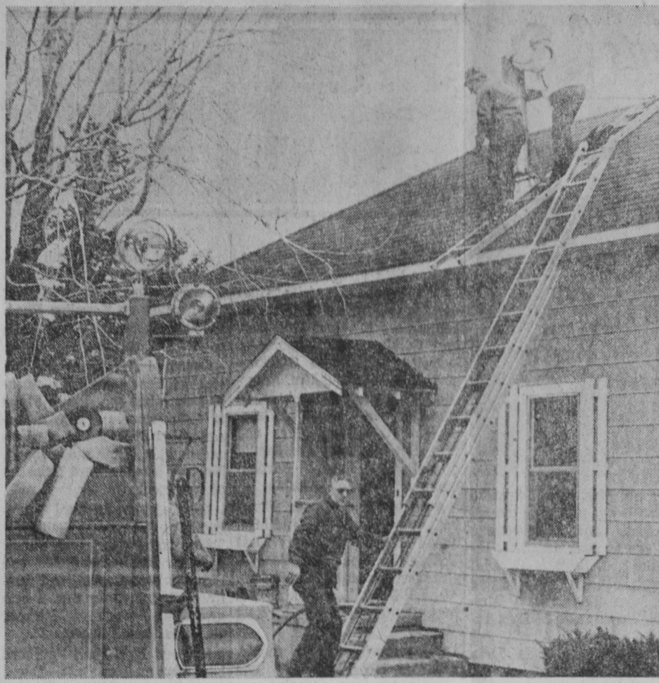
TAWAS CITY FIREMEN answered a call Monday afternoon at the residence of Mr. and Mrs. Kenneth Strobel on Harris Avenue. An overheated metal chimney connected to a wood burning stove caused the blaze. Fire damage was limited to the ceiling and attic area, although there was some smoke damage to the dwelling.—Tawas Herald Photo.
